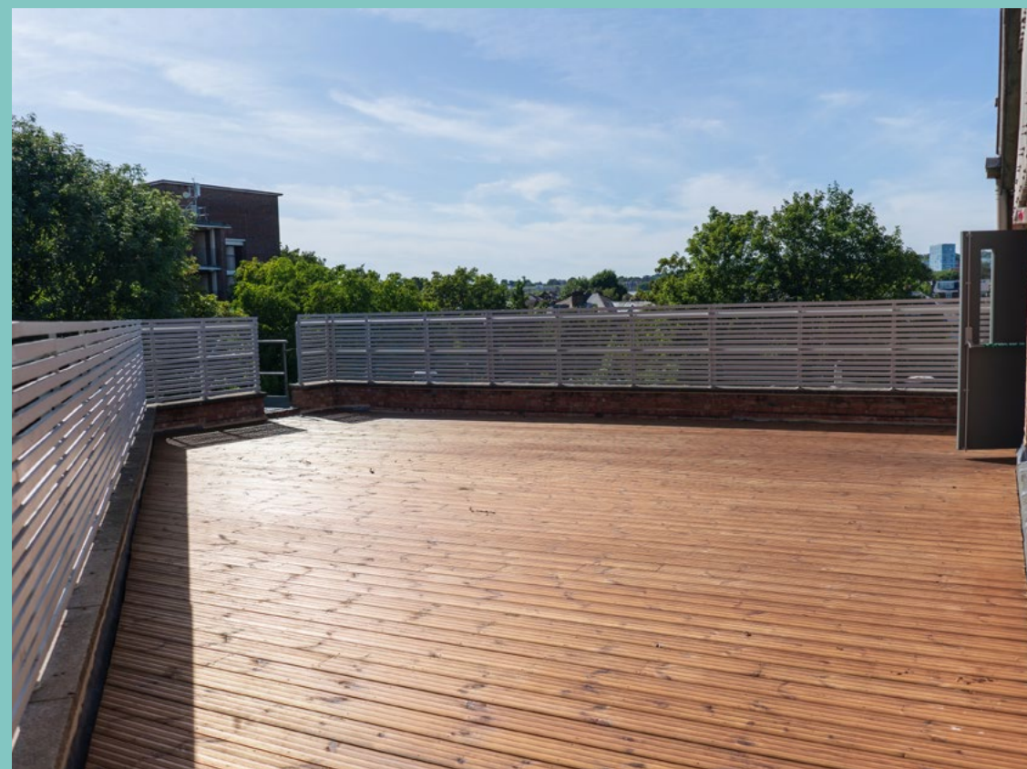
WAREHOUSE - 2ND FLOOR TERRACE
